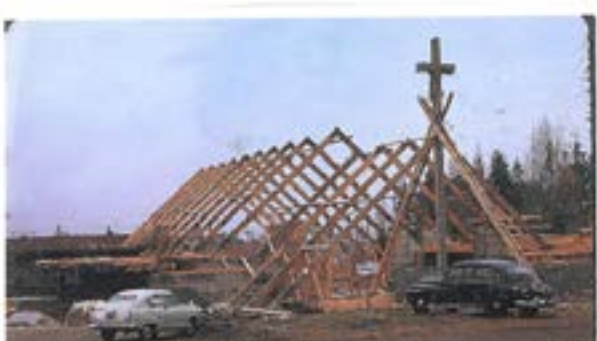
Church under construction in 1953
